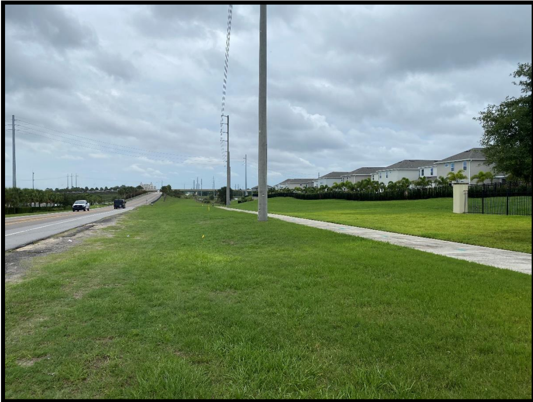
Photo 8: Old Lake Wilson right-of-way facing north
